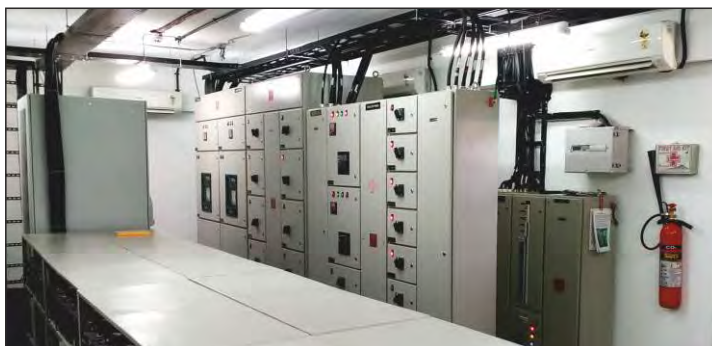
Power conditioning room for IUCAA Data centre with UPS, battery banks and control panels
