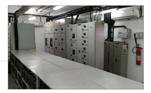
Power conditioning room for IUCAA Datacentre with UPS, battery banks and control panels
