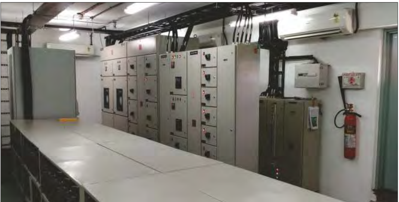
Power conditioning room for IUCAA Data Centre with UPS, battery banks and control panels (All Pictures are Credited to Shashank Tarphe, IUCAA)
