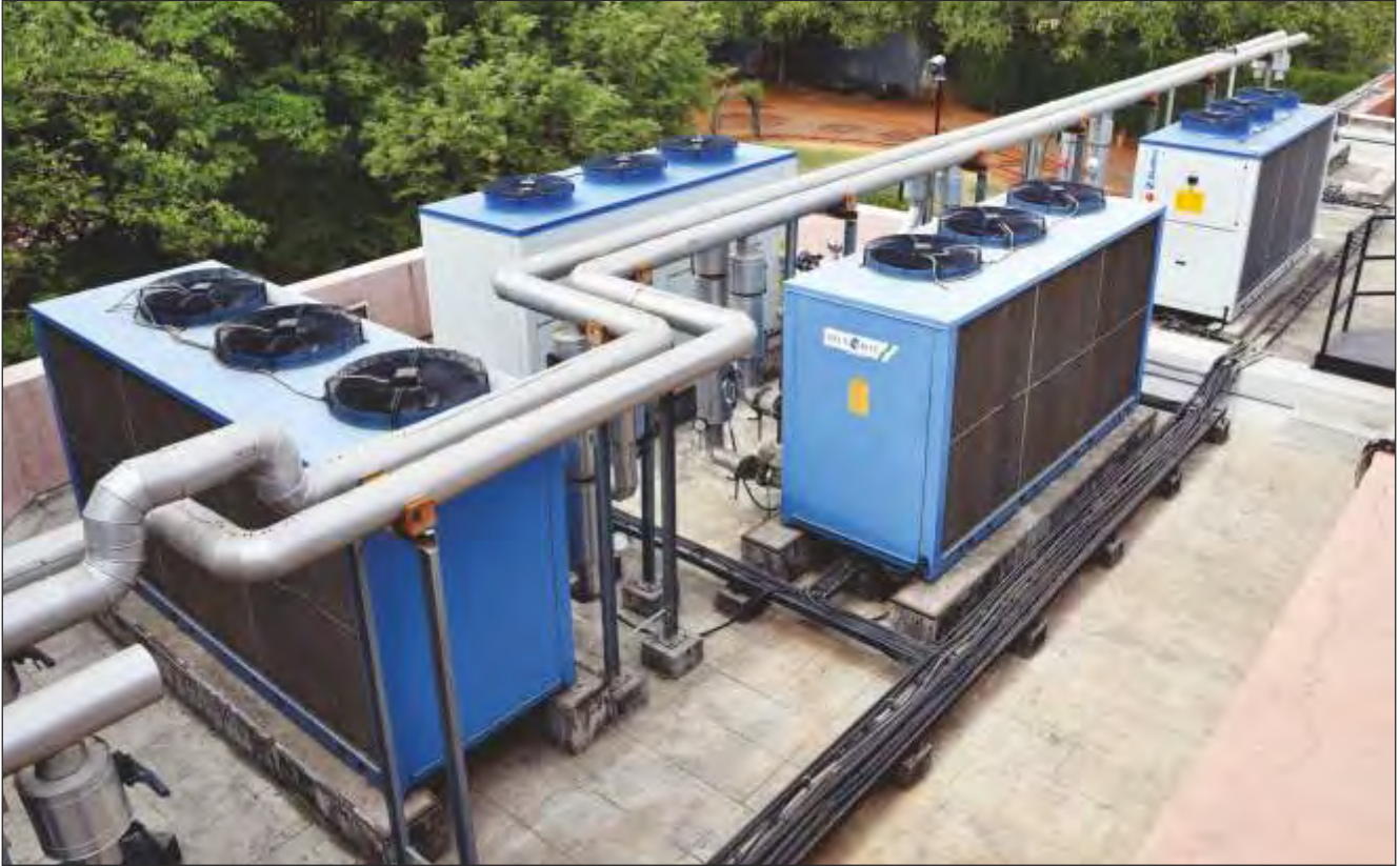
Chiller plant assembly for IUCAA Data Centre
