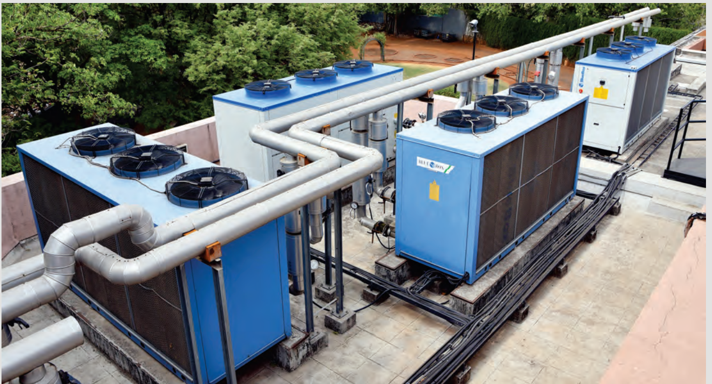
Chiller plant assembly for IUCAA Data Centre
