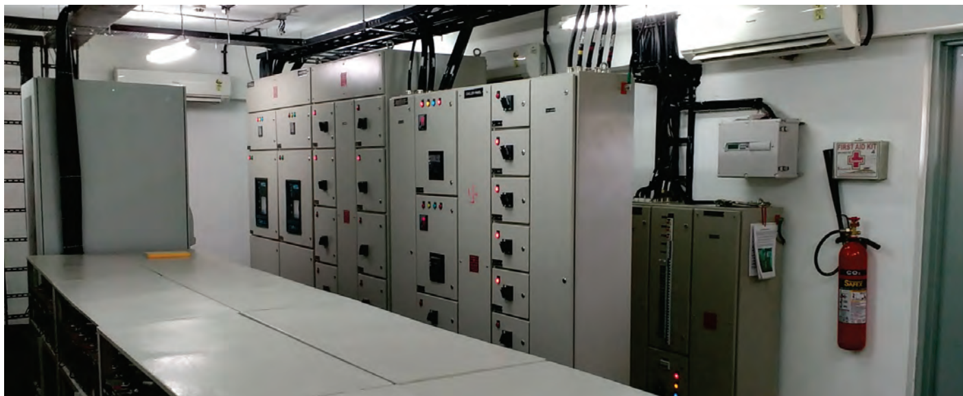
Power conditioning room for IUCAA Data Centre with UPS, battery banks and control panels
